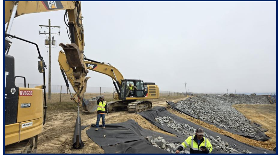
Fabric and Riprap Installation
