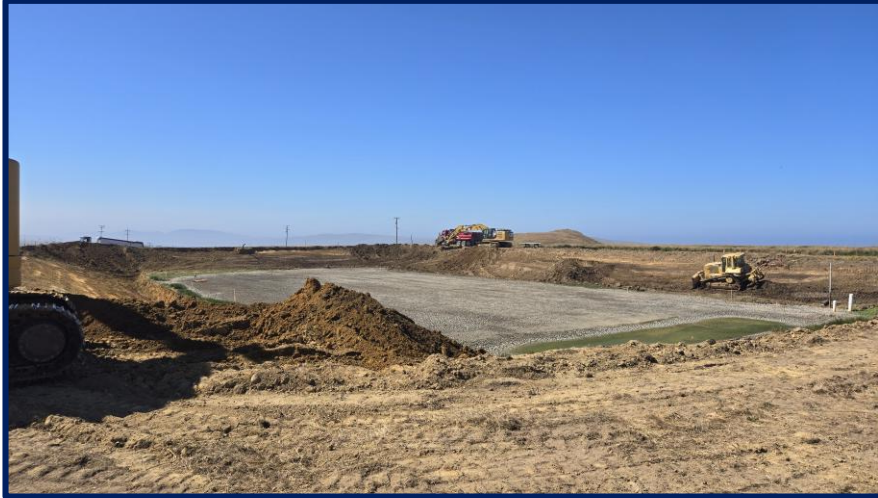
Storage Pond Slope Excavation
