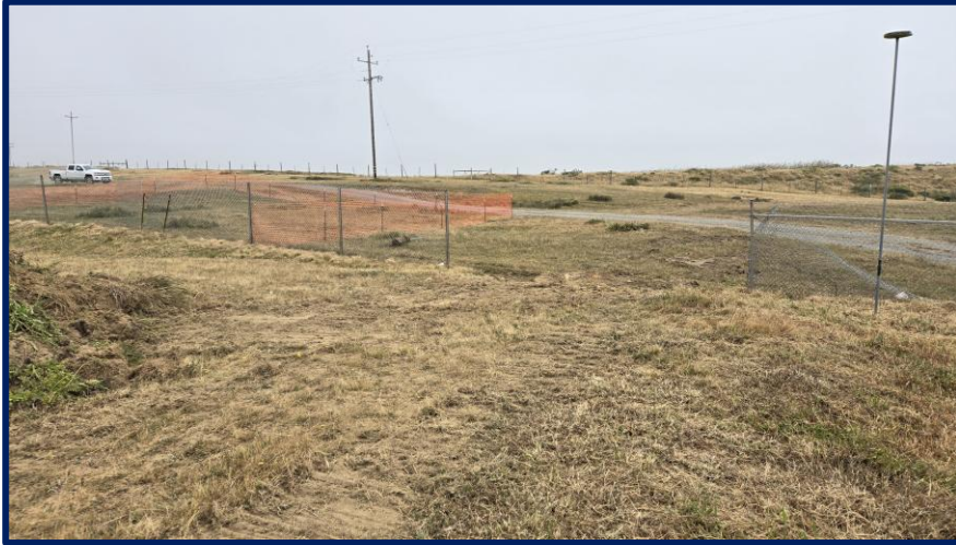
Wetland Protection and Temporary Construction Entrance
