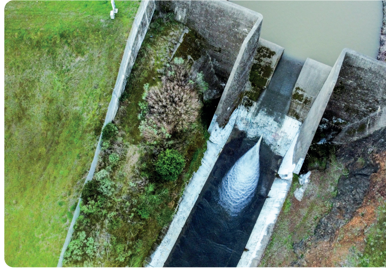
Stafford Dam spillway.
