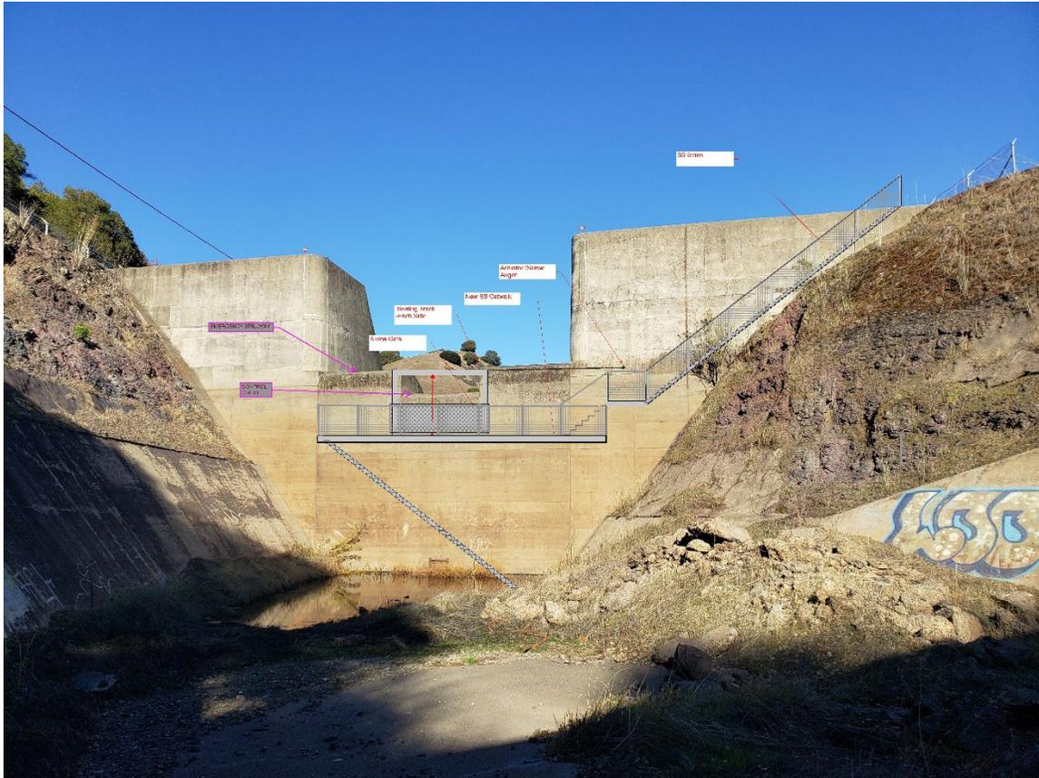
Figure 2. Dam spillway and proposed spillway modification
