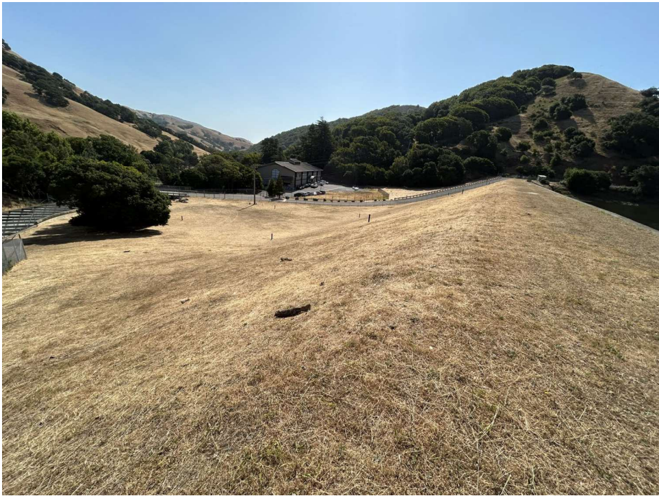
Photo 1: View of the downstream slope and crest observed from the left end of the dam.
