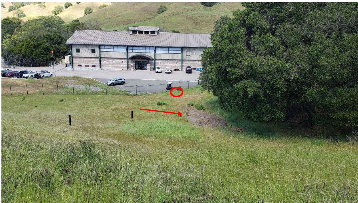
Photo 4: Partial view of the downstream slope and right groin. The arrow points to the location of the perforated collection pipe installed adjacent to the blanket drain. The outfall is near the toe, just south of the parking lot (circled).
