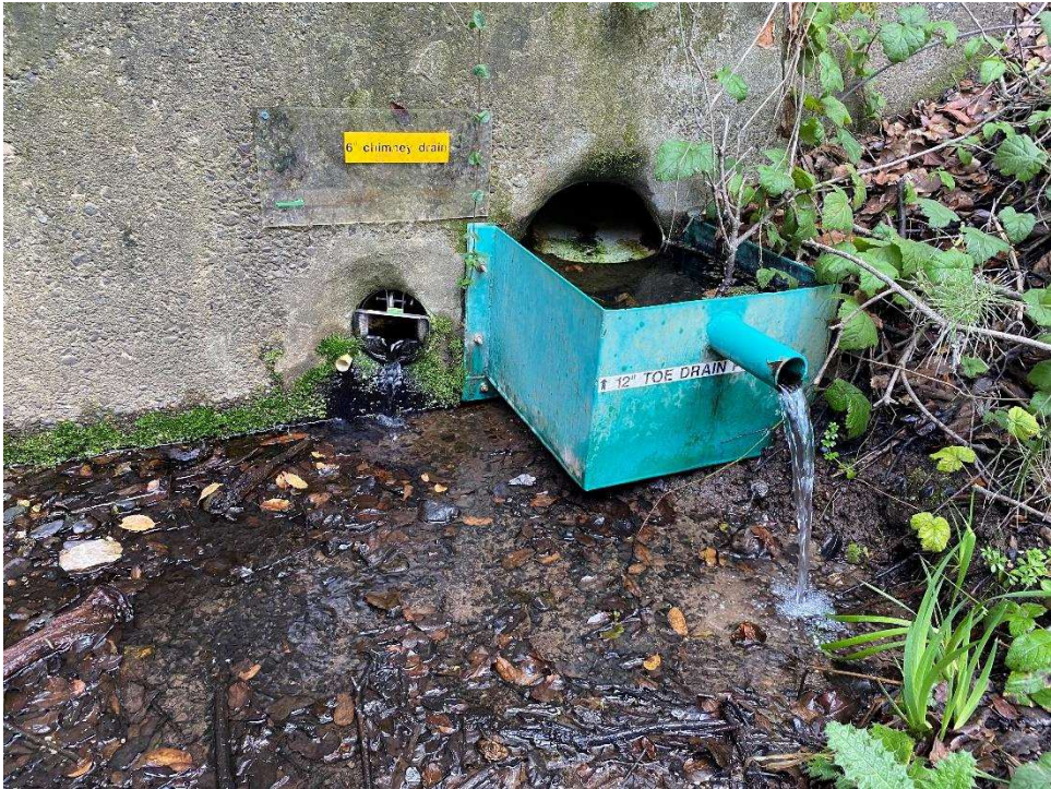
Photo 6: Outfalls for the 6-inch chimney drain (left) and the 12-inch toe drain (right).
