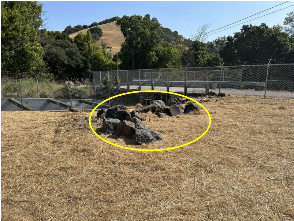
Photo 10: Remove the remaining stones from the downstream toe (in yellow circle).
