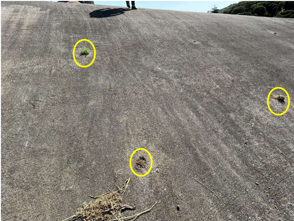
Photo 7: Clear vegetation in the weep holes along the upstream face (in yellow circles).
