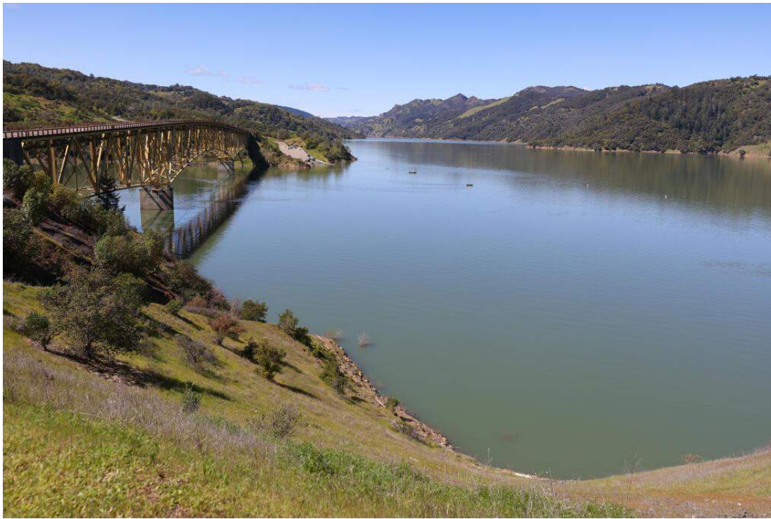
The Warm Springs Creek Bridge over Lake Sonoma, Tuesday, March 26, 2024. (Christopher Chung / The Press Democrat)
