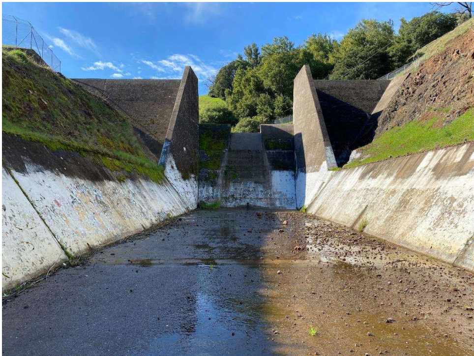
Photo 4: The ogee overpour and spillway chute was free of debris and in satisfactory condition.
