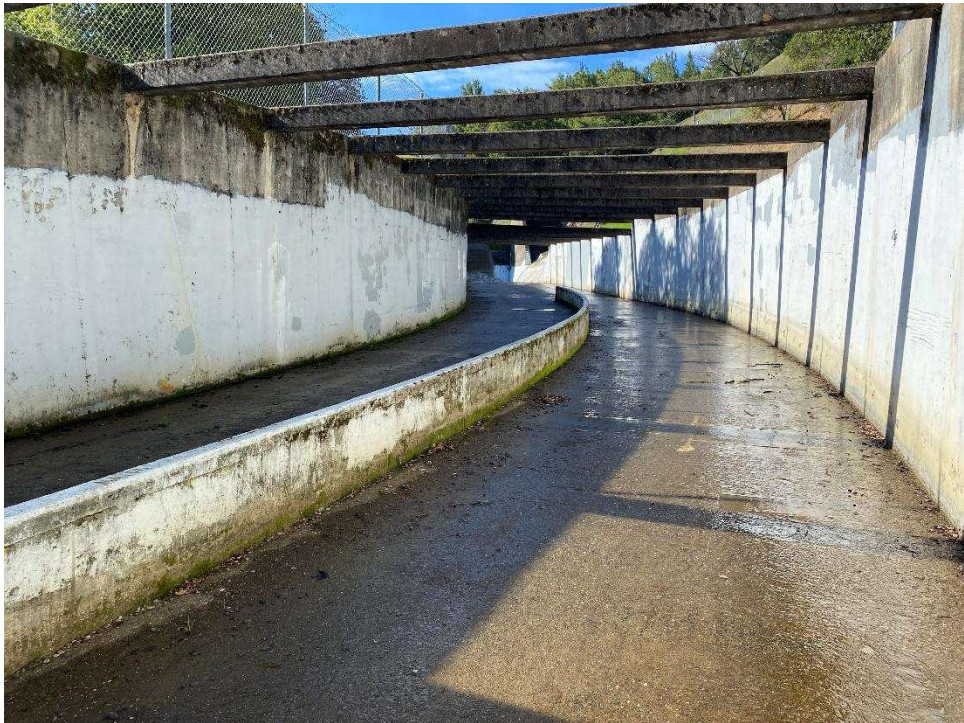
Photo 3: Spillway chute was clear and in satisfactory condition. Vegetation above the spillway had been removed since the last inspection.
