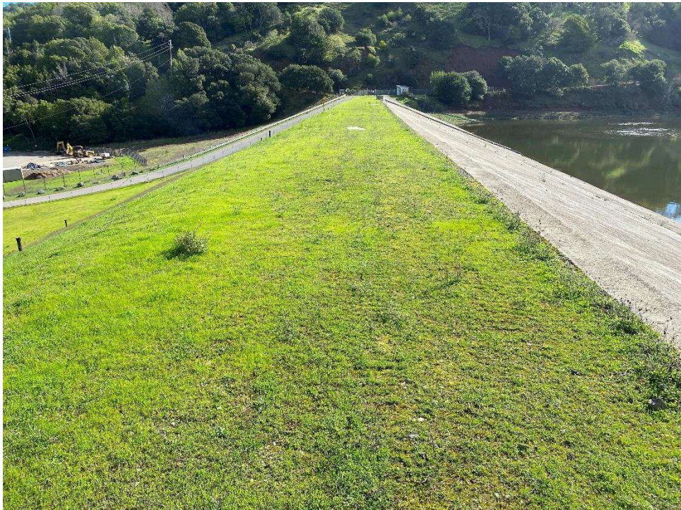
Photo 1: Dam crest looking from the left abutment towards the right.
