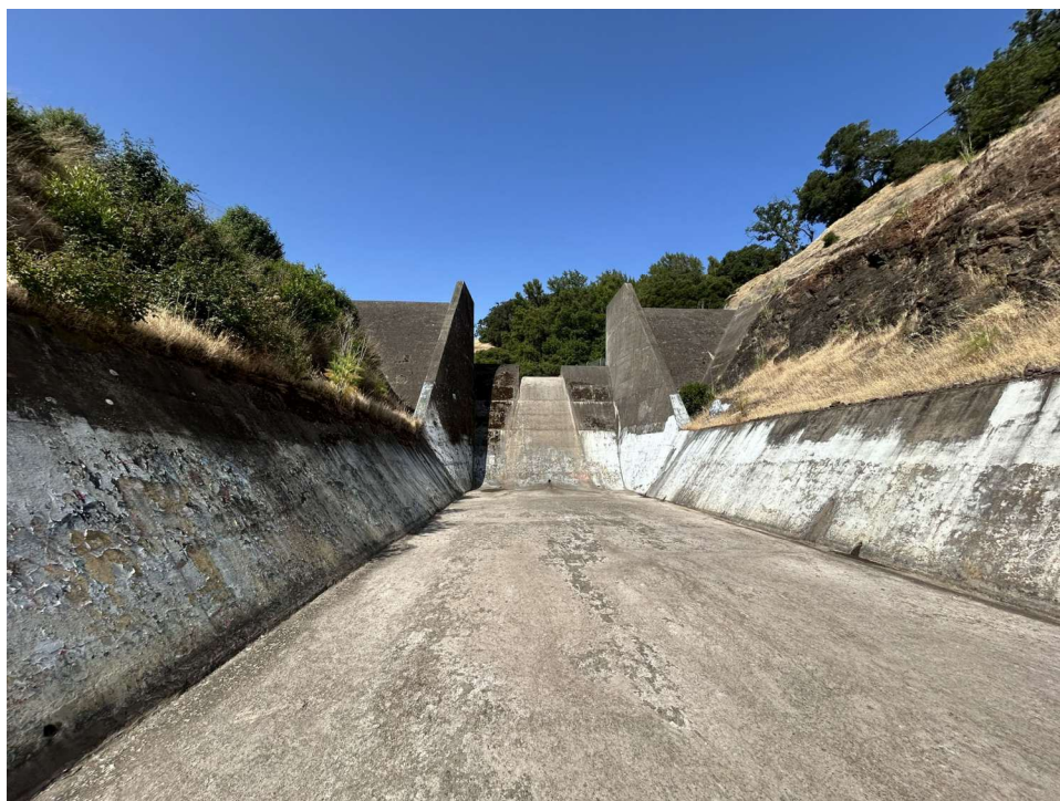
Photo 3: View of the ogee overpour and concrete spillway chute looking upstream.
