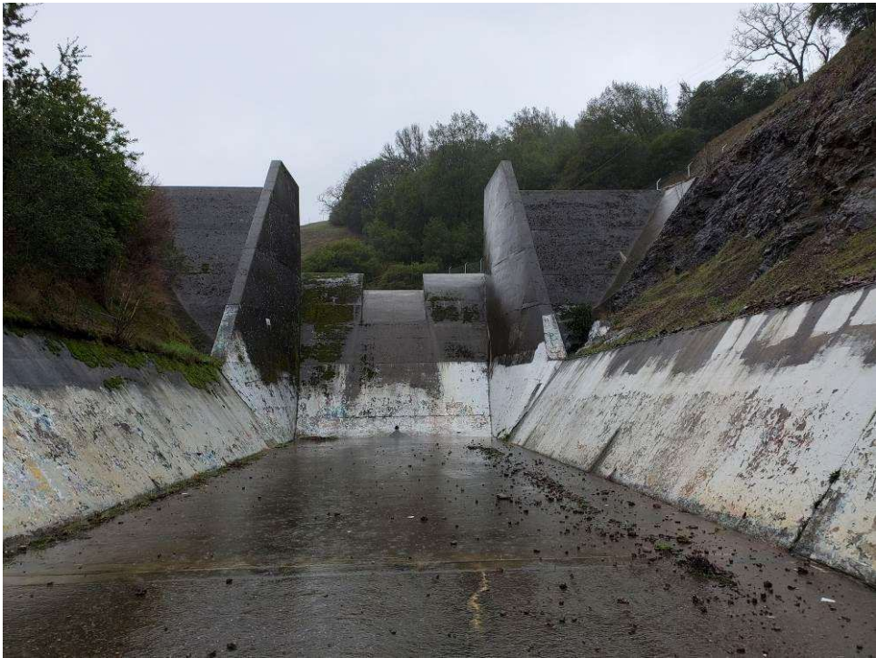
Photo 2: View of the ogee overpour and concrete spillway chute.
