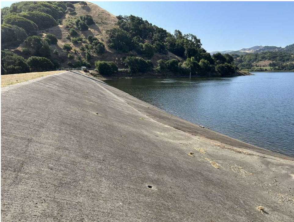
Photo 2: View of the upstream face observed from the left end of the dam.
