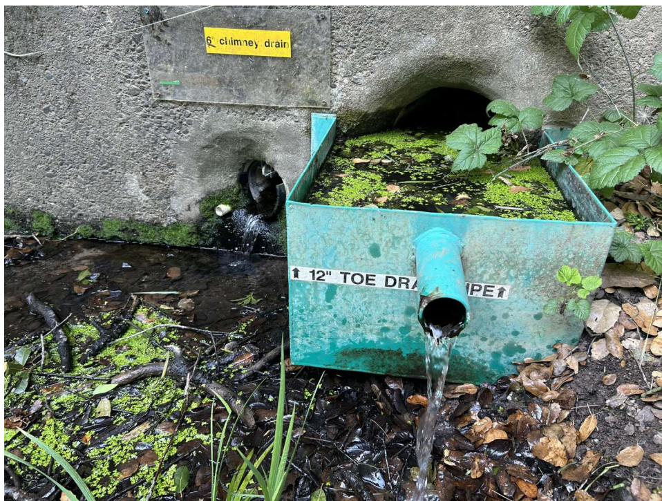
Photo 4: View of the outfalls for the 6-inch chimney drain (left) and the 12-inch toe drain (right).
