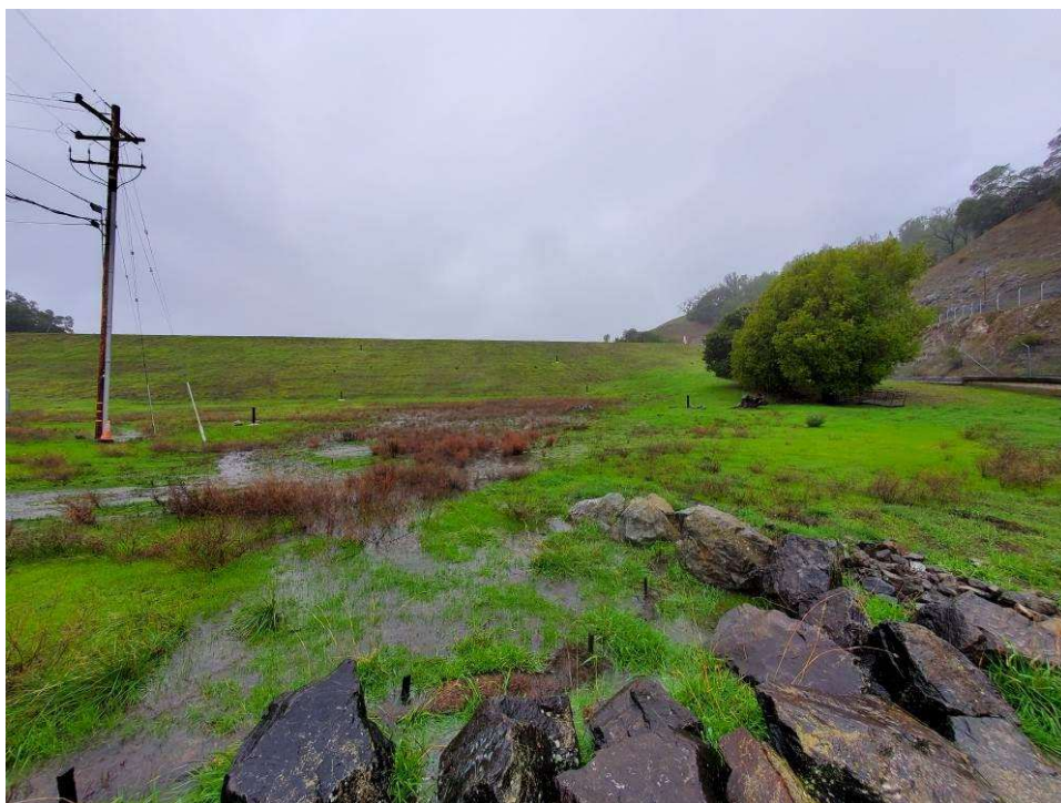
Photo 6: View of the runoff at the downstream toe of the dam.
