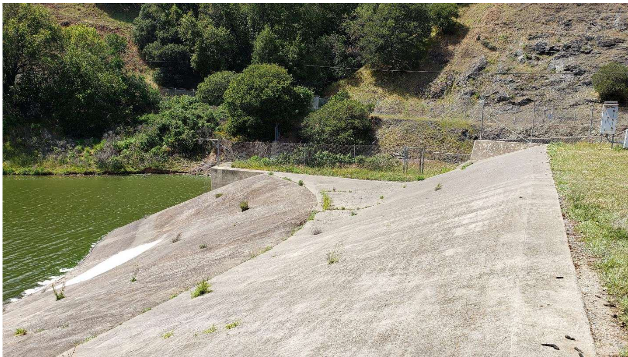
Photo 2: The spillway entrance at the left end of the dam was unobstructed.
