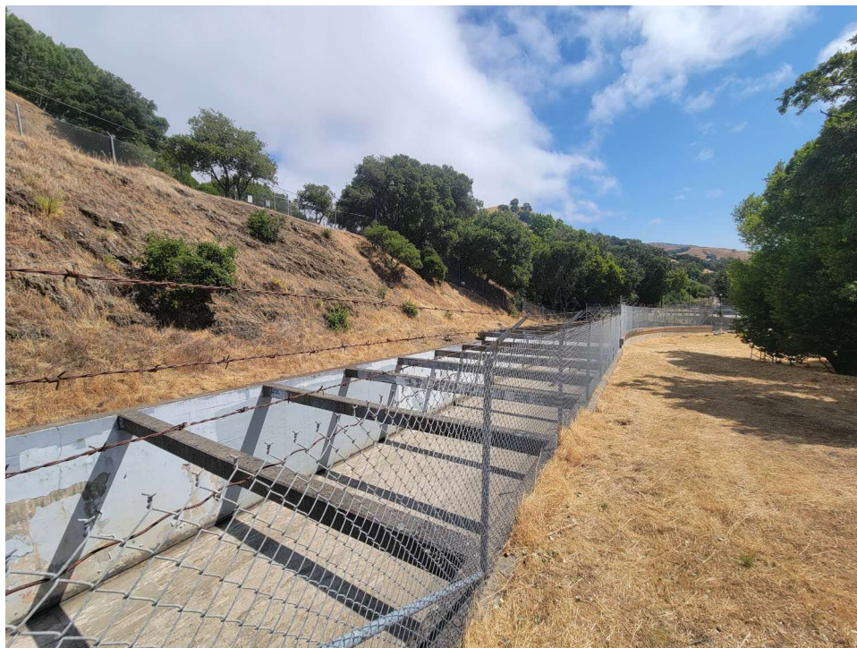
Photo 13: Photo provided by the owner on 6/25/25 of the recently removed overhanging vegetation along the spillway channel walls.
