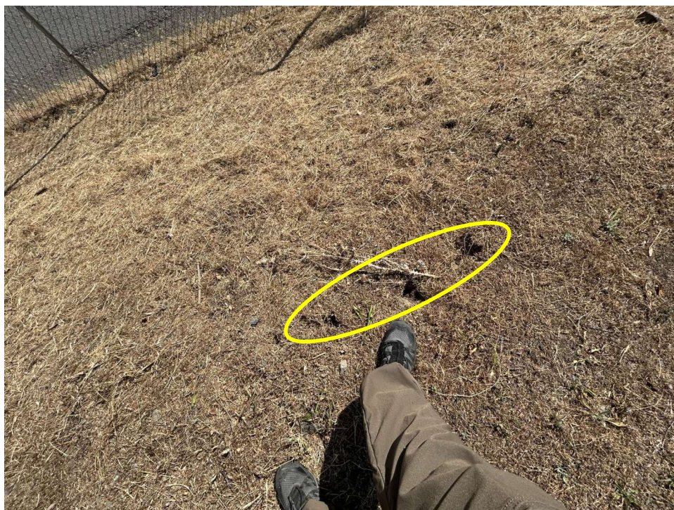
Photo 12: Breakup, backfill, and compact existing rodent burrows (in yellow circle).
