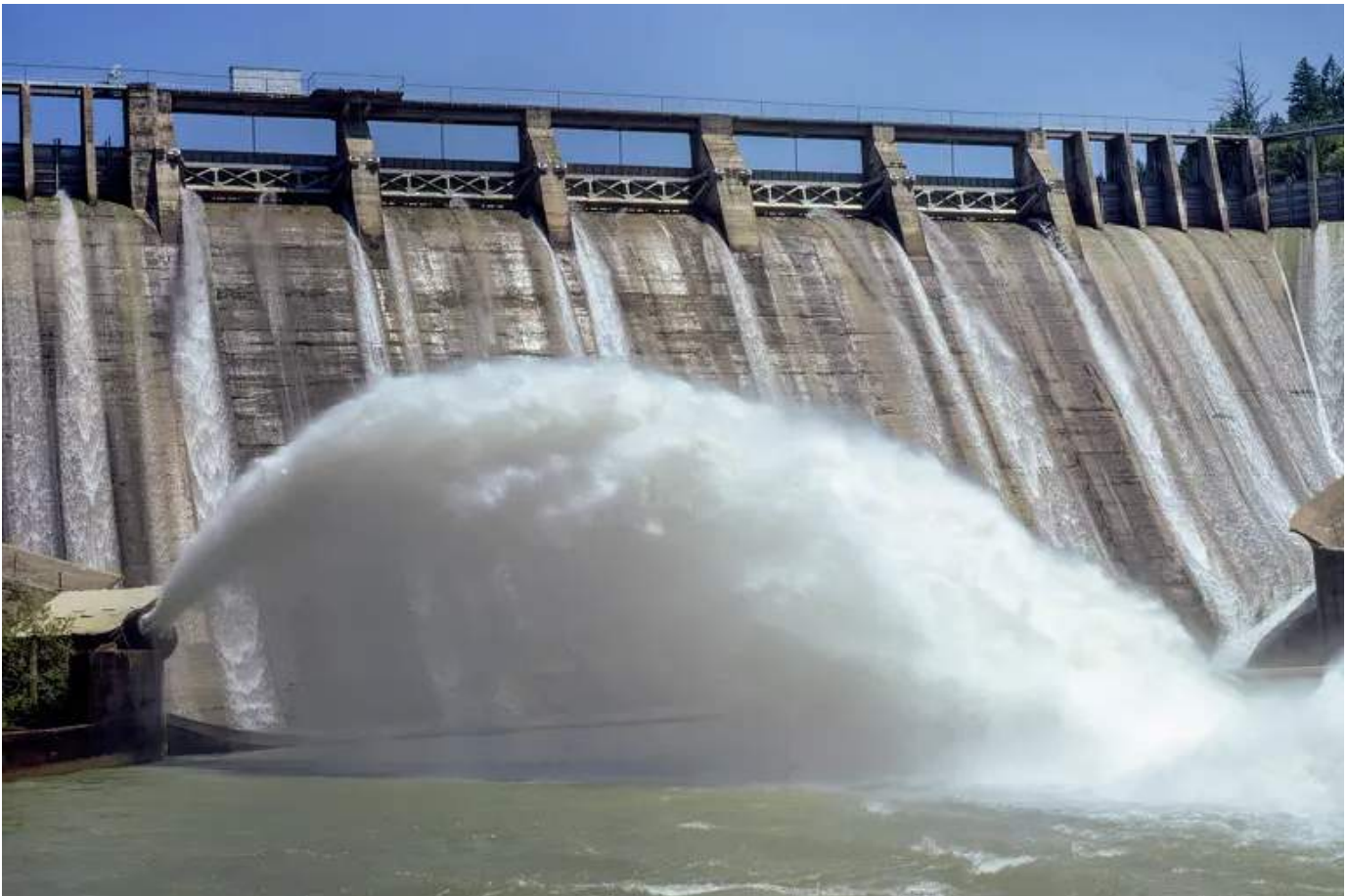
A water release from the concrete Scott Dam, built in 1922, on the Eel River within Lake County, Calif. The dam was originally constructed as a source for electricity and owned by Pacific Gas & Electric. Photo taken May 26, 1967.
