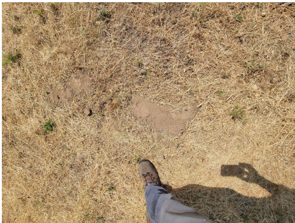
Photo 14: Photo provided by the owner on 6/25/25 of the recently broken up, backfilled, and compacted rodent burrows on the right downstream groin.
