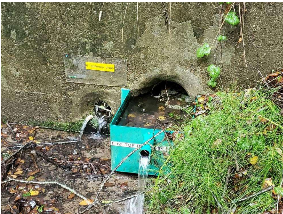
Photo 7: View of the outfalls for the 6-inch chimney drain (left) and the 12-inch toe drain (right).
