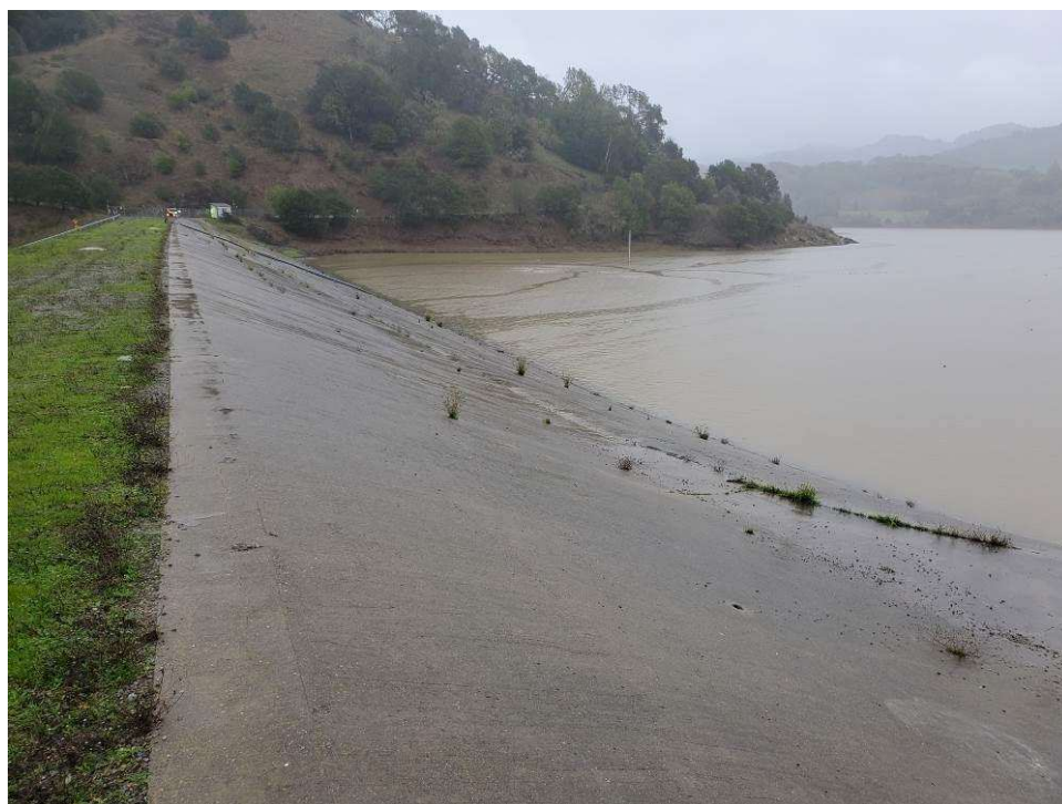
Photo 1: View of the upstream concrete liner from the crest on the left side of the dam.
