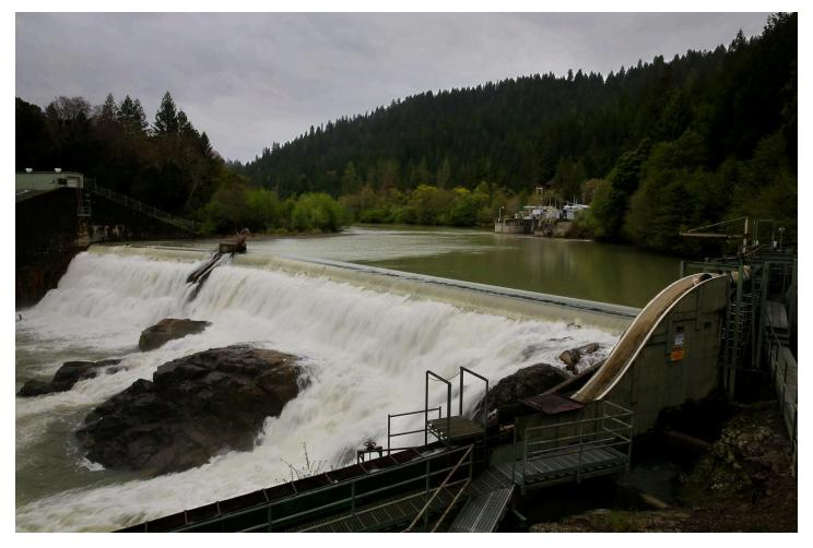
Water from the Eel River collects at the Van Arsdale Reservoir and flows over the Cape Horn Dam. A percentage of the water is redirected through a diversion tunnel, at the building in the background, to the Potter Valley Powerhouse and east fork of the Russian River. Christopher Chung — The Press Democrat
