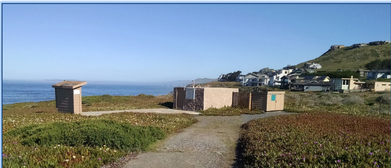
Oceana Marin Pump Station
