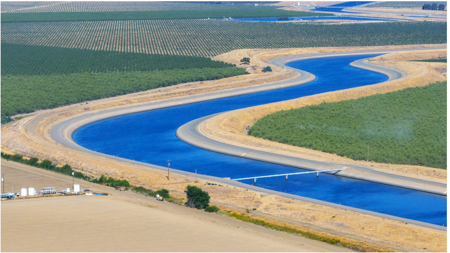
The California Aqueduct near Highway 165 in Los Banos, Merced County, on Sept. 25, 2024. Brian van der Brug — Los Angeles Times
